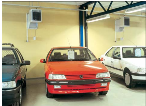
Mixing cabinets combine heating and ventilation. The mixing cabinet saves energy by mixing return air with fresh air in individually preset proportions.
